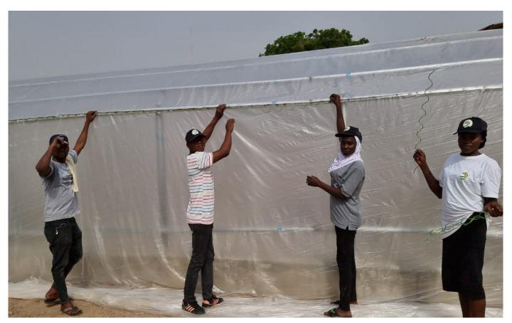
EBAFOSA trained youth taking roles in building a solar dryer to help avert post harvest losses from the local community. The solar dryers are an inexpensive tools built to help drying of cereals and other leguminous produce. The drying allows the farmers to later add value to their produce and increase their shelf life.
